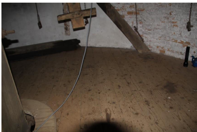
Herstelde houtendelen kapzolder.
